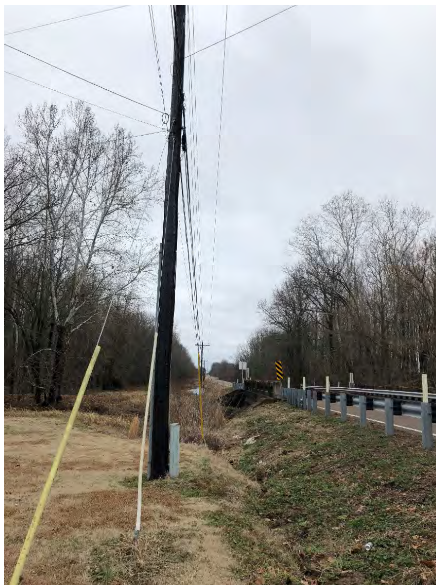
Existing Utility Pole on North Side of Bridge
