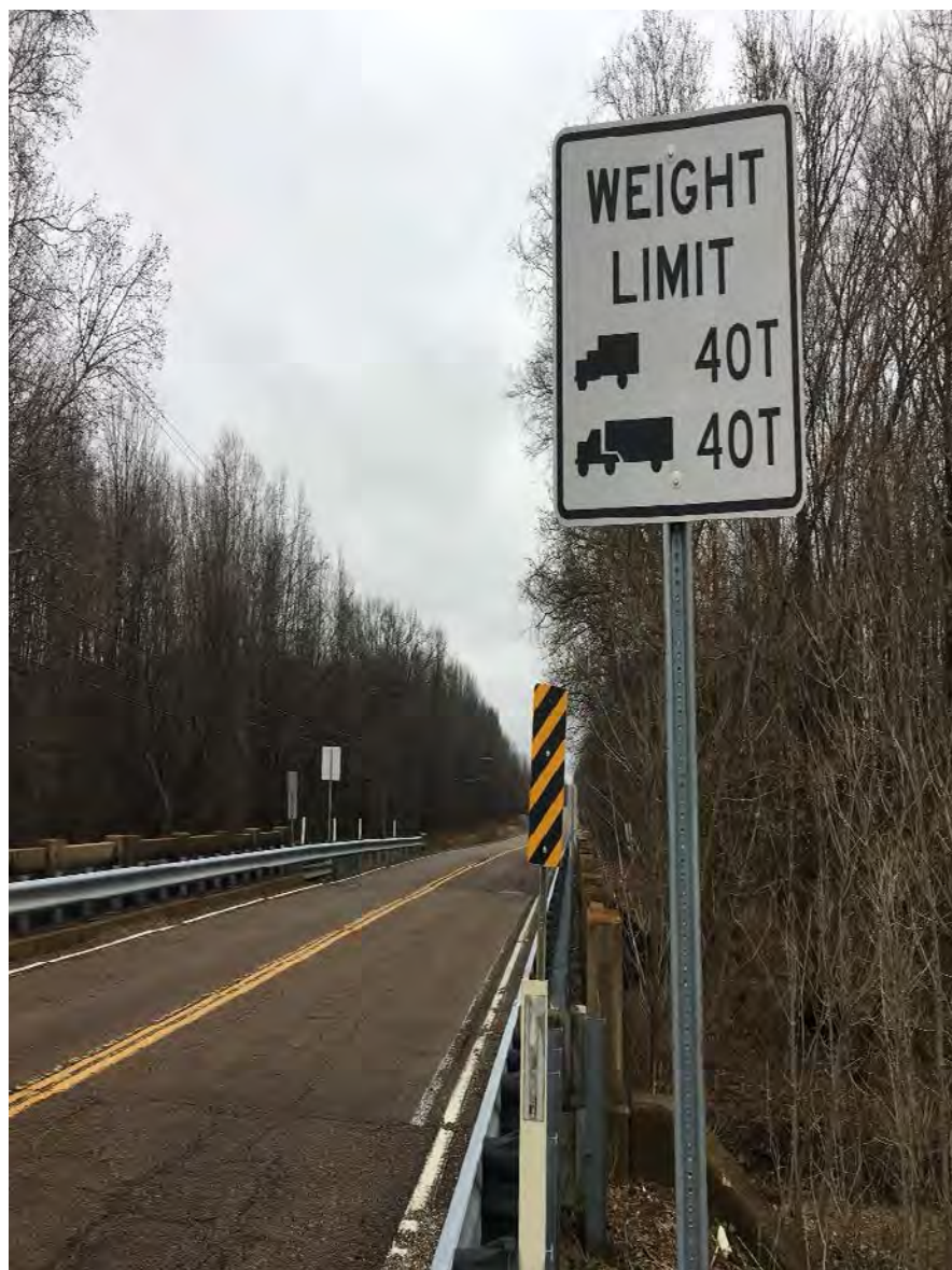
Weight Limit Sign at West Approach
