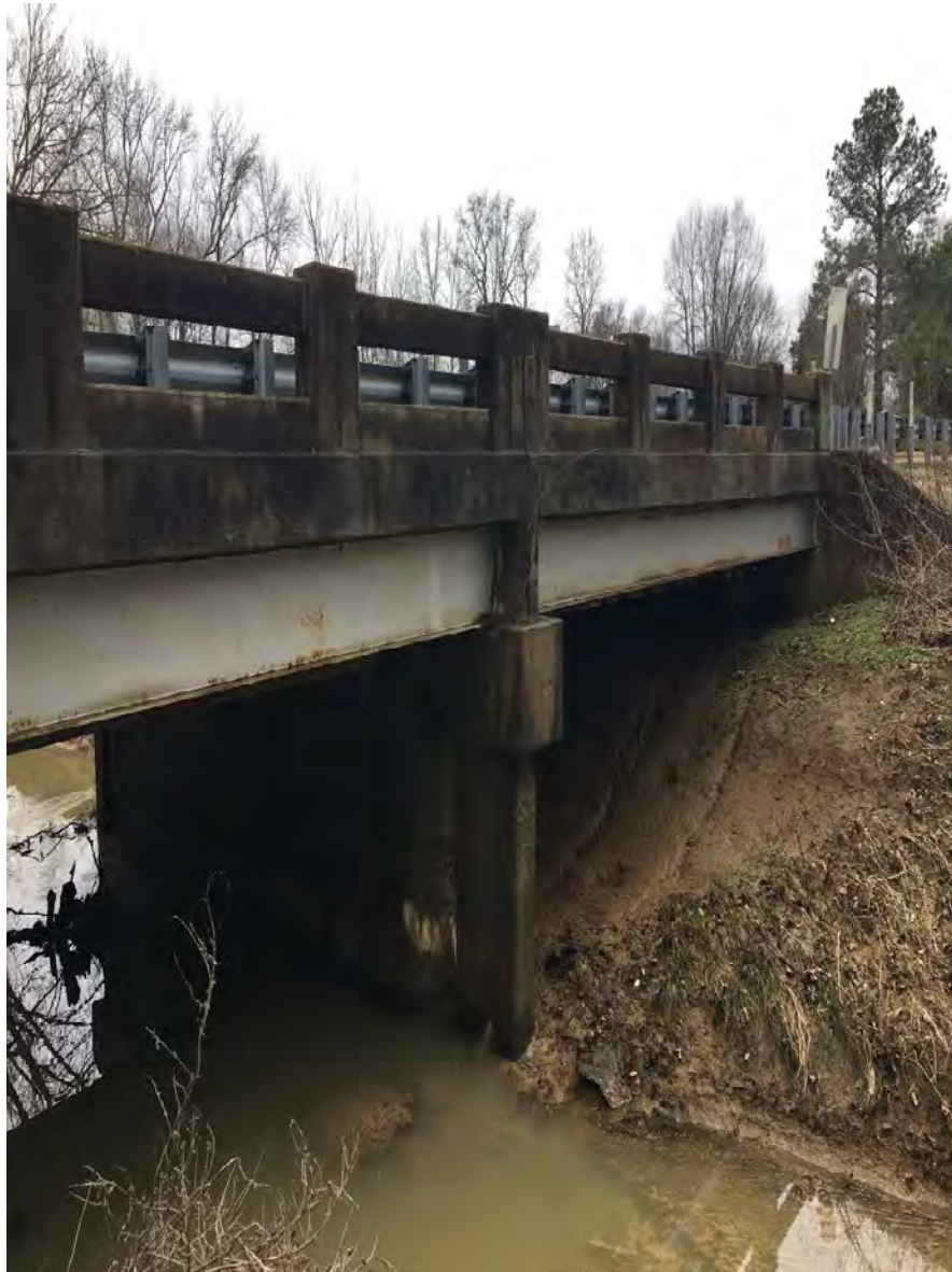
Outlet Pier from East Bank
