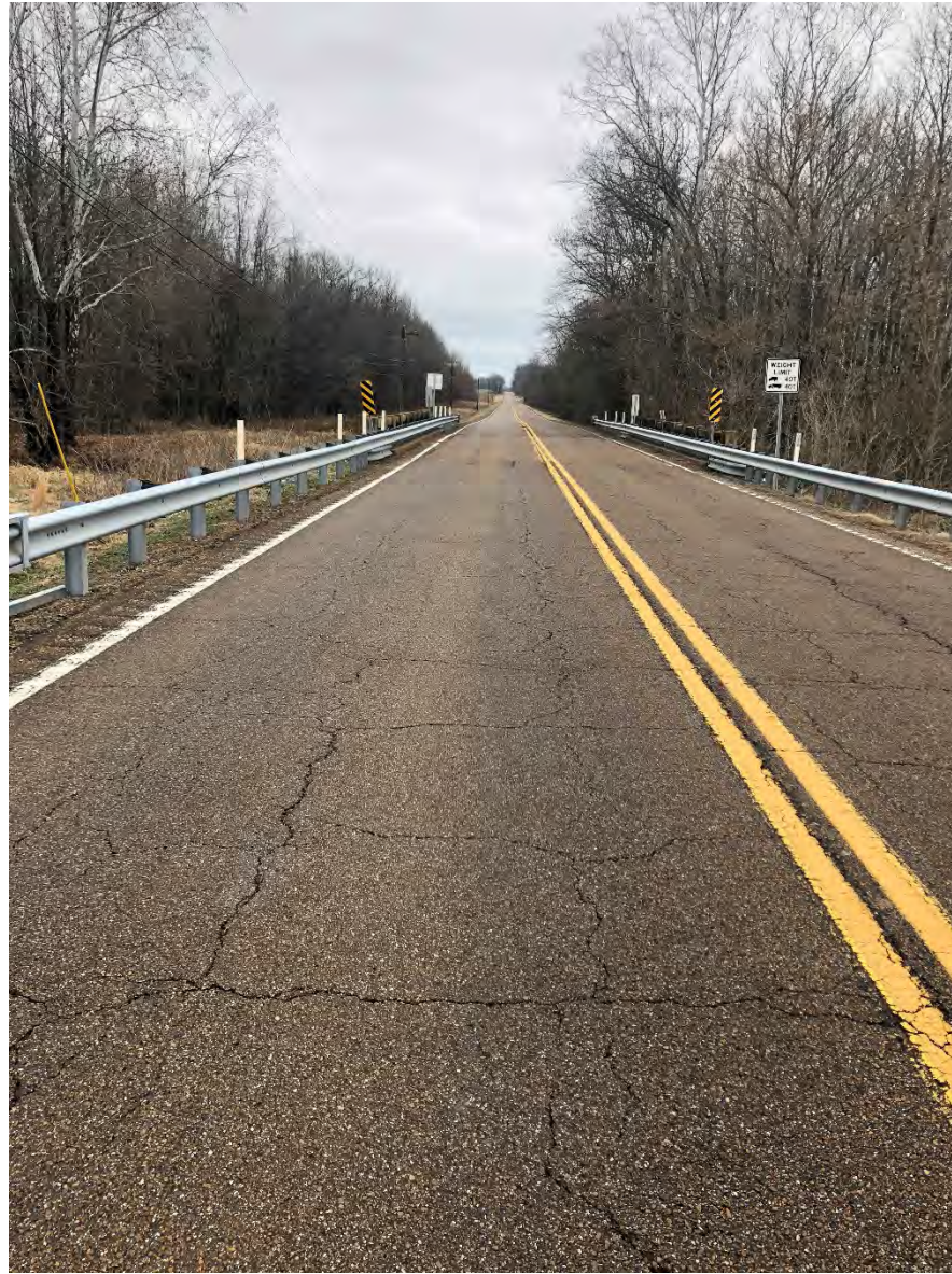
Eastbound Approach of Bridge
